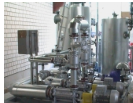
Flash vessel installed on-site
